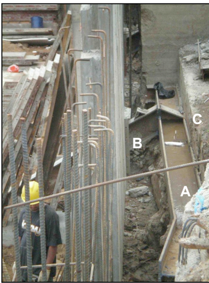
Walers (A) and rakers (B) protected subway vault (C) during excavation.
